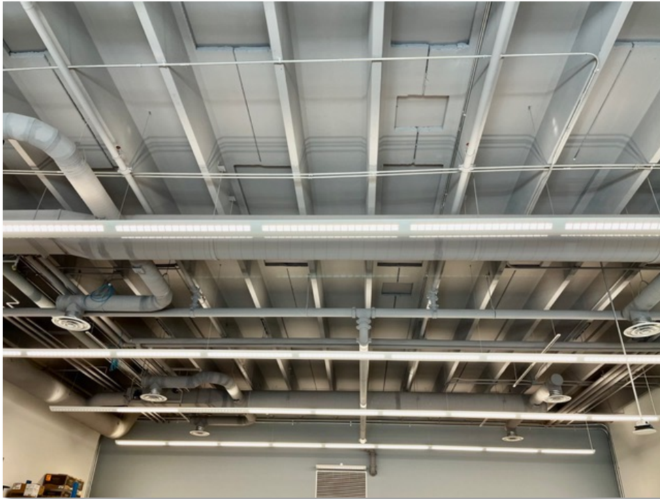
Double "T" precast roof construction
