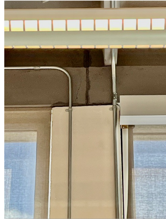
precast edge beams over columns
